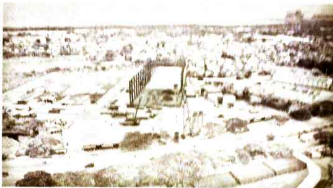
Piling works on the Light Rail Transit Line 1 Cavite extension began last Sept. 1. (COMPASS HANDEUT)
